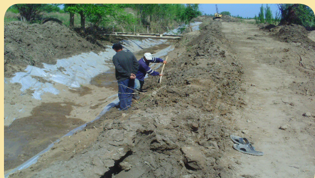
Picture 4. Laying ground
