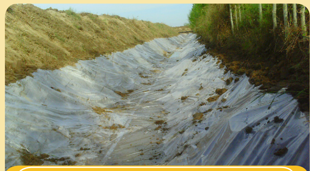
Picture 3. Placing film
