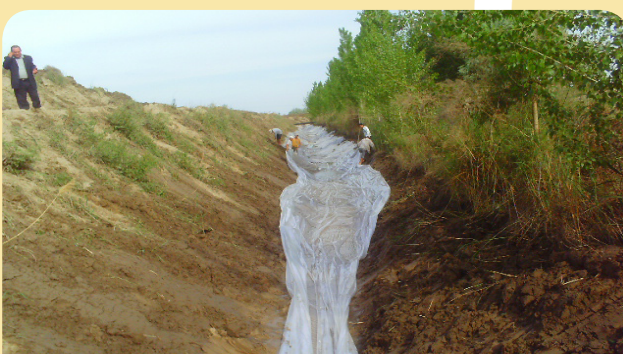
Picture 2. Placing film
