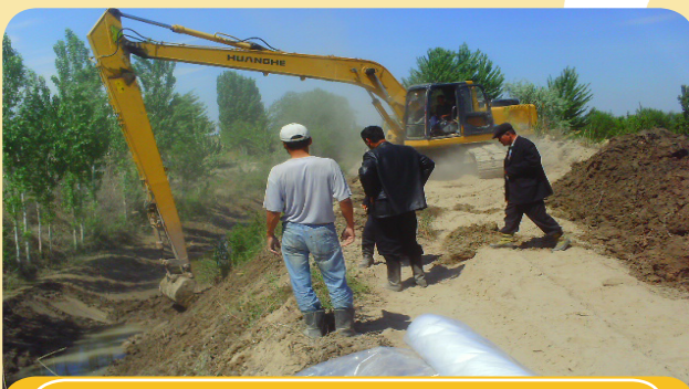
Picture 1. Cleaning of the canal
