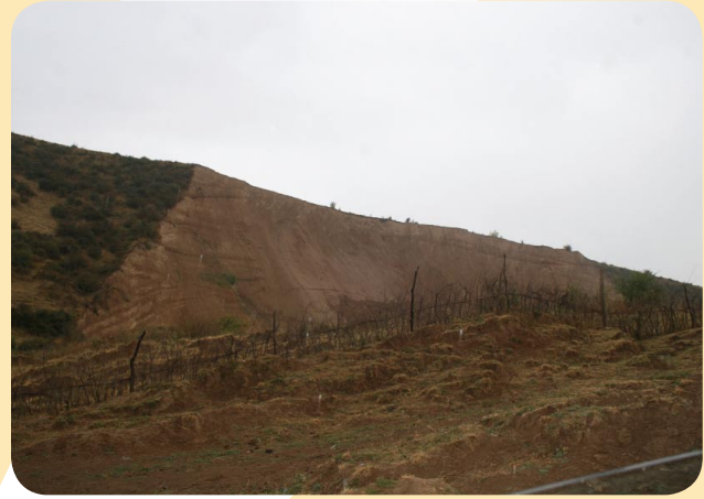
Photo 18. A landslide in the surroundings of mountain settlements in Tashkent province
